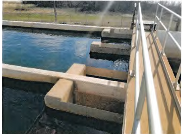
Olney Water Treatment Plant (2022)
